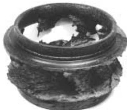
Figure 1. Erosion of grey cast iron impeller after two months handling coal dust
