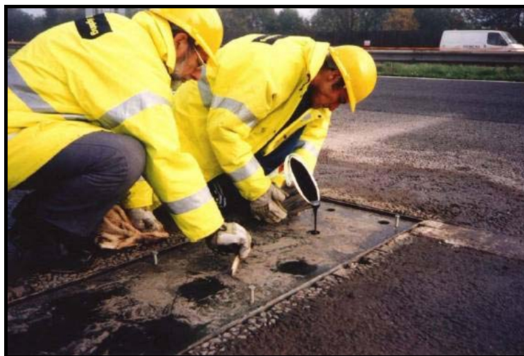
Figure 5.2.1.2.6.1 Constructing an embedded load sensor
