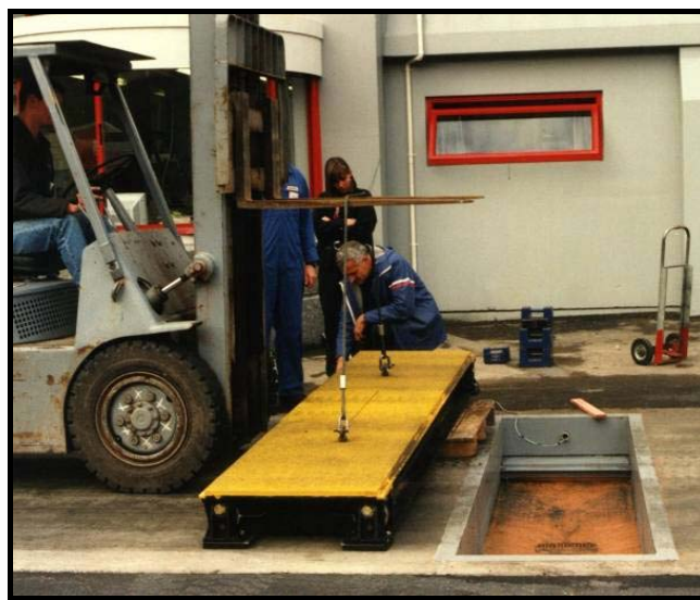
Figure 5.2.1.2 Typical construction of a fixed axle weighbridge
