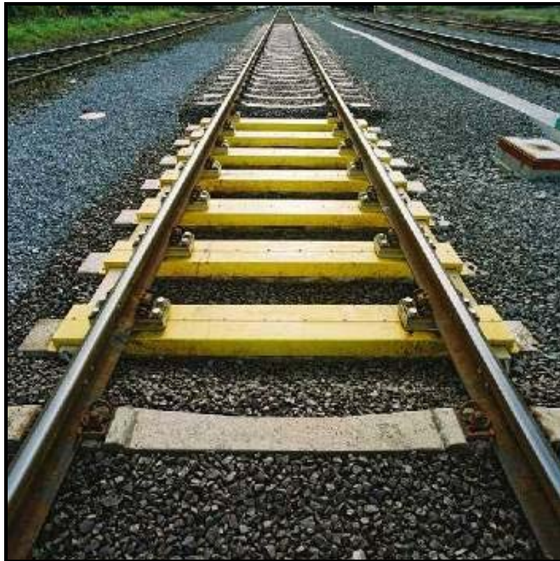
Figure 5.2.2.7 Active sleeper weighbridge
