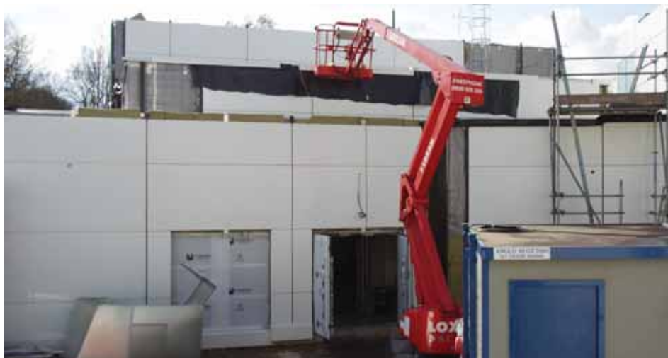
The new linac building, construction nearly complete
