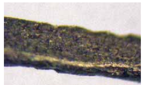
Strand damaged by wear and corrosion
